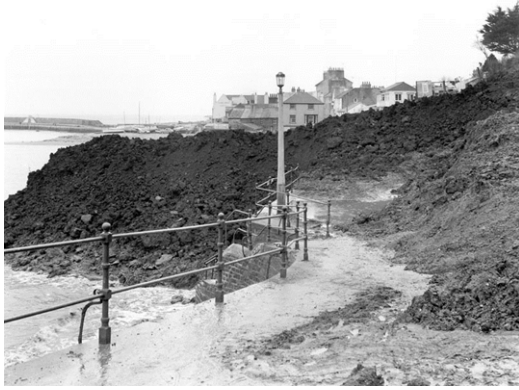
Figure 1.4 Coastal erosion, 1962 (image courtesy of Environment Agency)
